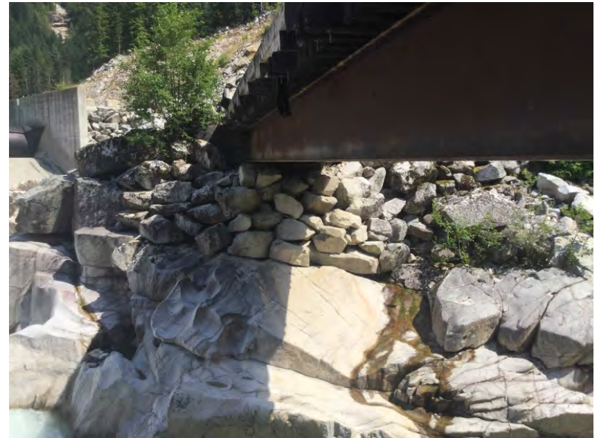
Left Bank Abutment
