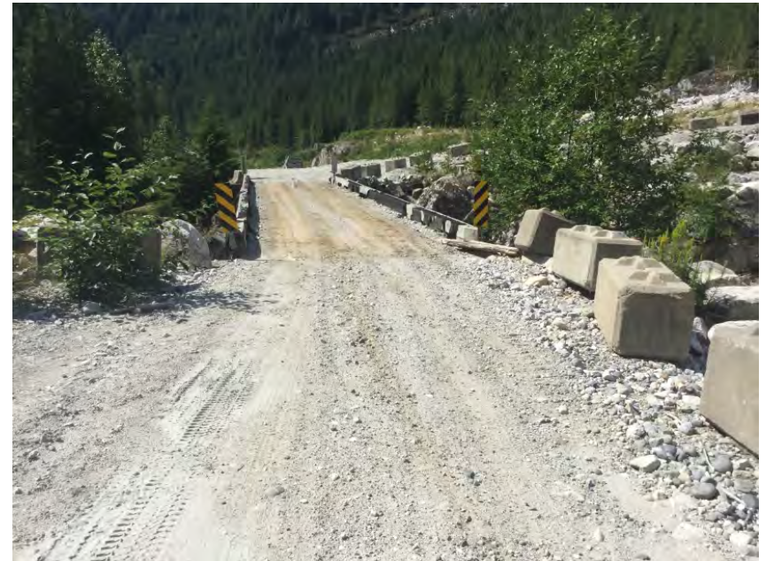
Left Approach Facing Bridge
