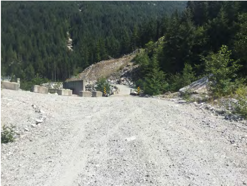
Right Approach Facing Bridge
