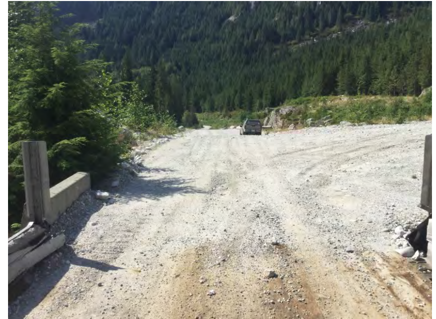
Right Approach Facing Away From Bridge
