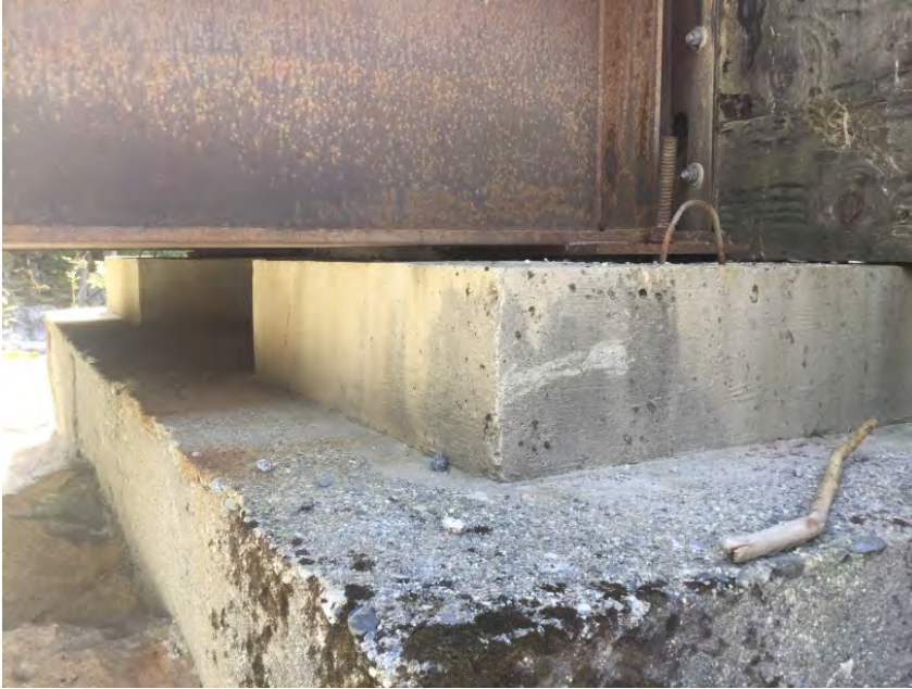
Right Abutment Upstream Girder
