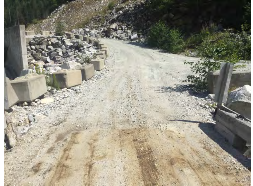
Left Approach Facing Away From Bridge
