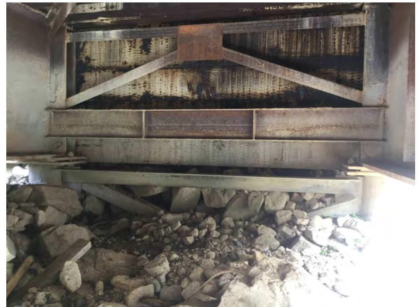
Left Bank Abutment
