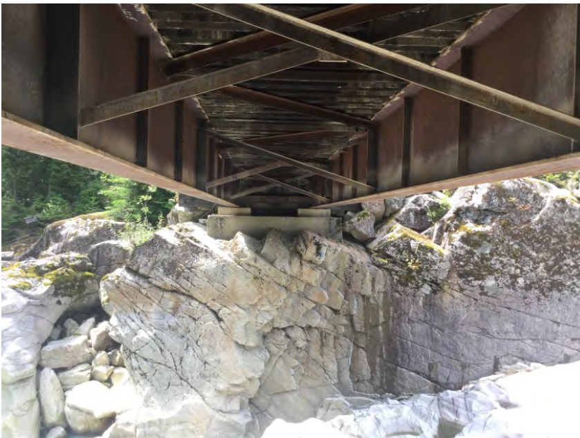
Right Bank Abutment
