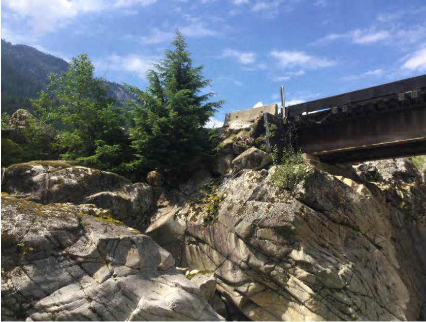
Short Fender with Steep Drop at Right Approach Downstream Corner
